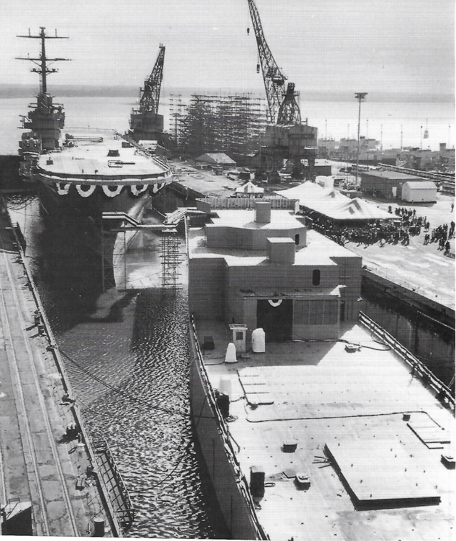
Facing above Commissioning the amphibious assault ship Sumter , 14 December 1969. The Sumter , along with the amphibious command ship Blue Ridge , commissioned in 1970, marked the end of new ship construction at the Philadelphia Navy Yard. Temple University Urban Archives.
