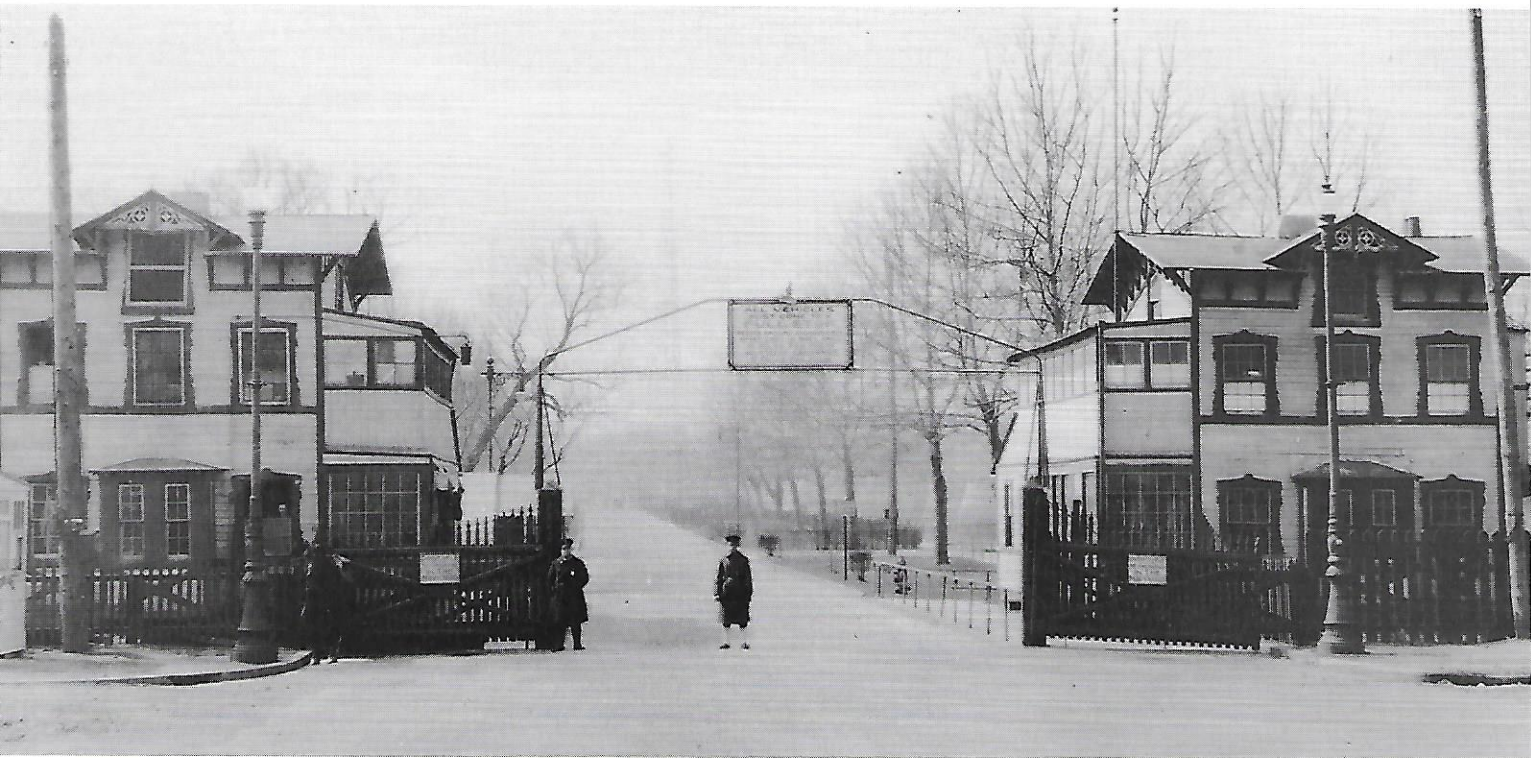
The main gate on Broad Street before its removal in 1926 to make way for a new gate for the Sesquicentennial Exposition. NARA Washington, D.C., Still Picture Branch.
